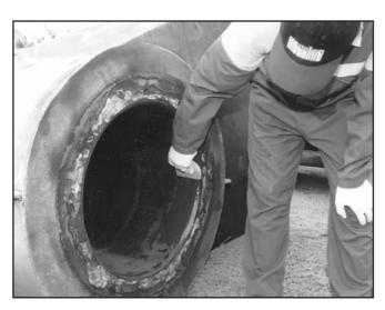
FAST NEWMETAL is an extremely fast curing repair epoxy putty that contains a blend of specially graded ceramic particles. This results in an inert high density material that provides exceptional properties when used on equipment exposed to erosion, cavitation, corrosion and chemical attack. It is especially suited for use in emergency repair applications or where very low application temperatures are prevalent.
