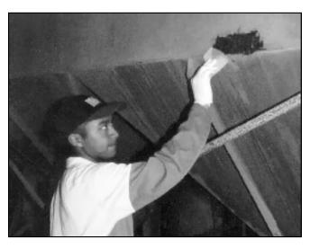
FASTPATCH is technically advanced, fibre reinforced fast curing repair putty suitable for patching gaps and repairing holes that are difficult to bridge. It contains unique high strength fibres, specially selected to provide increased resistance to pressure and impact allowing emergency repairs to be carried out that resist harsh service conditions. It also cures at very low temperatures to provide a tough inert repair. TYPICALLY USED ON:
